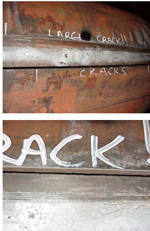
Figure 3-10: Container with crack through keyway, probably caused by overheating. A larger radius may help eliminate this problem
