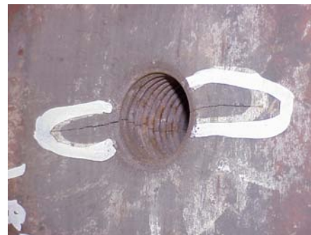
Figure 3-8: Container cracked through hole for lifting eye. Container was also overheated. (Photos courtesy of Lake Park Tool)
